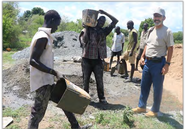
Lynn Kandel overseeing the construction of a new school
