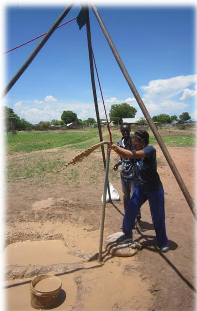
"It's a tough job!" Leisa using Jim's locally-manufactured well-digging tools.
