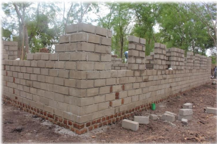
Construction progress in Pochalla
