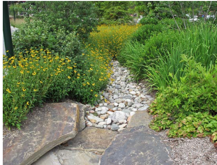
Water is directed to a detention basin along a path of river rock lined with attractive native species. Shoemaker Green, University of Pennsylvania, Philadelphia, PA.
