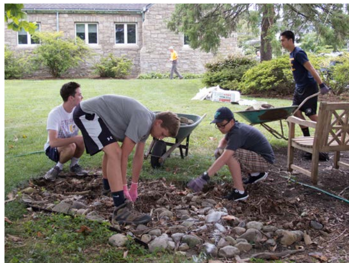
Members of Boy Scout Troop 219 from Wayne, PA began the process of installing the rain garden by removing the river-rock around the outflow pipe that brings water across the courtyard.
