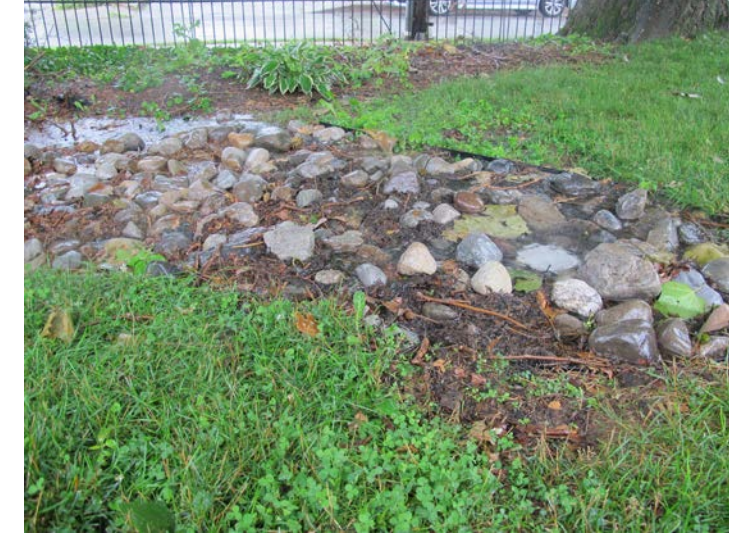
An unsightly rock pile marked the spot where stormwater ran to the edge of the property, often flooding the sidewalk before finding a storm drain.
